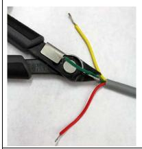
Cut off the green cable not necessary using pliers.
