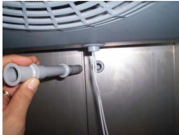
Below you can see the components of the drain pipe.
