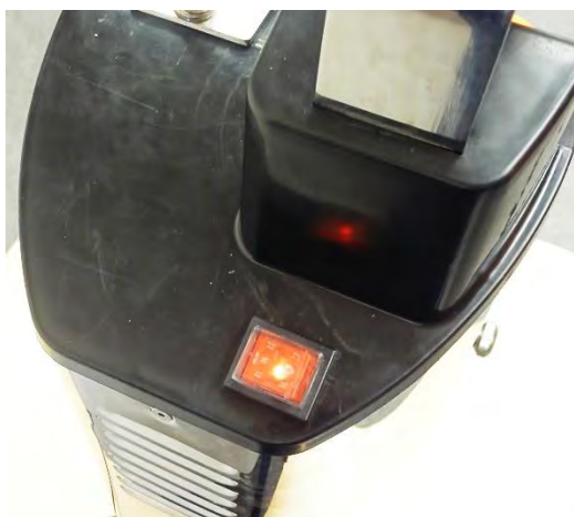
Picture 7: main switch
